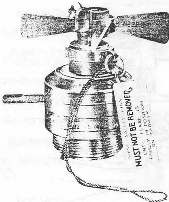
Figure 147—Nose Fuze No 288 Mk III
