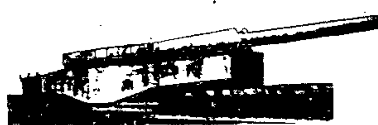
310 mm GLOTT GUN, MOUNTED ON 280 mm RAILWAY GUN [28 cm K 5 (E)] MOUNT
